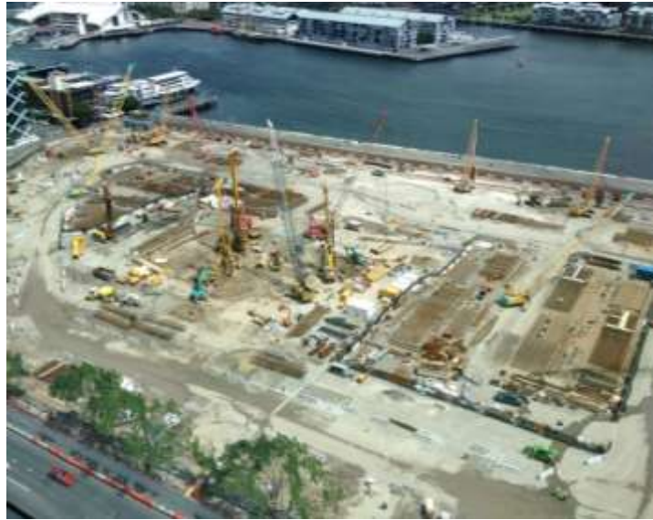
Barangaroo site under construction (photo by author, 07/03/2012)
